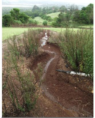
Figure 6 – Existing Scoured Drainage Line below Pipe under Terranora Road
